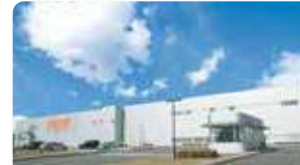
2006 Yamazaki Mazak Manufacturing Corporation, Minokamo Plant 2 (Japan)
