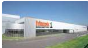
1983 Yamazaki Mazak Manufacturing Corporation, Minokamo Plant 1 (Japan)
